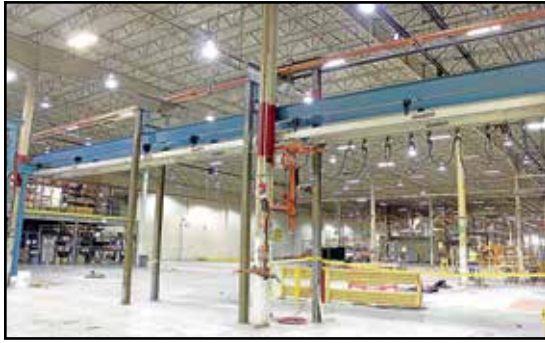
1,000 LB KNIGHT UNDERSLUNG DOUBLE GIRDER CRANE SYSTEM
